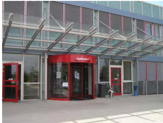
Main Entrance to Building F
